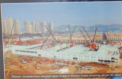
Picture : Wuoshenshan Hospital takes shape in Wuhan, Hubei province, on Jan 30, 2020
